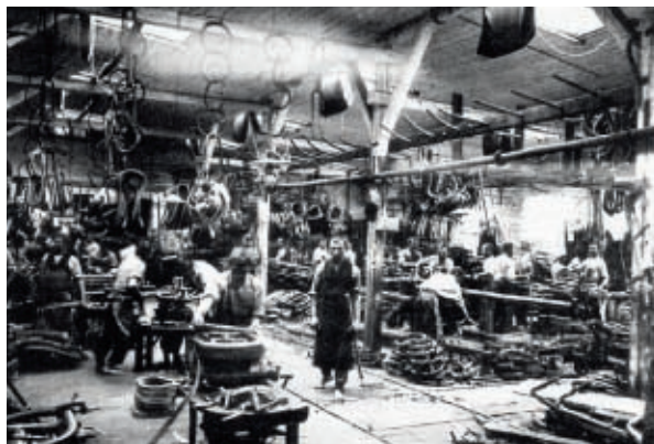
THONET FABRIK IN BYSTRITZ // THONET FACTORY IN BYSTRITZ
